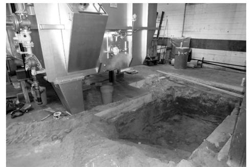
The furnace base and furnace are installed and work has begun on the run-off pit.
