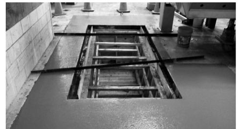
The completed run-off pit with the forms still in place.
