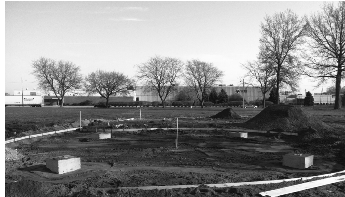
The footings and form for the park's shelter pad.
