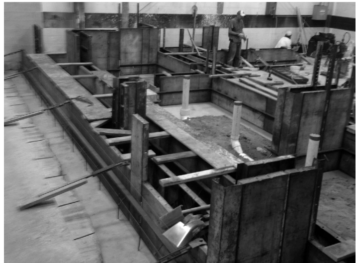
Formwork is completed and ready for the final concrete placement.
